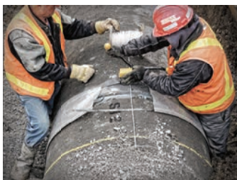
Diaper is placed around the joint and straps are tightened
