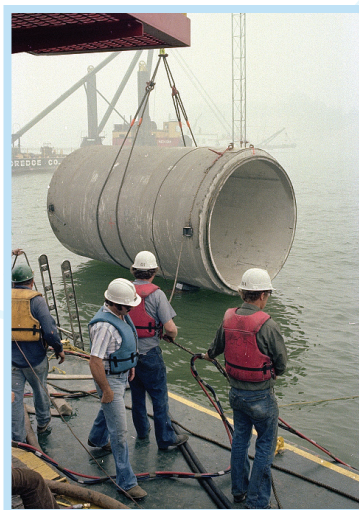
Subaqueous joint installation lugs are clearly visible on this pipe.
