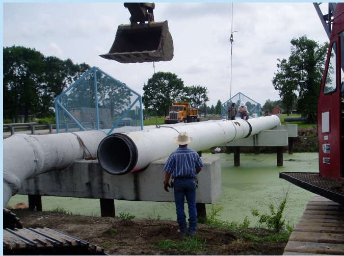
Multiple lengths of Concrete Pressure Pipe can be welded together to extend span length and reduce the number of piers.
