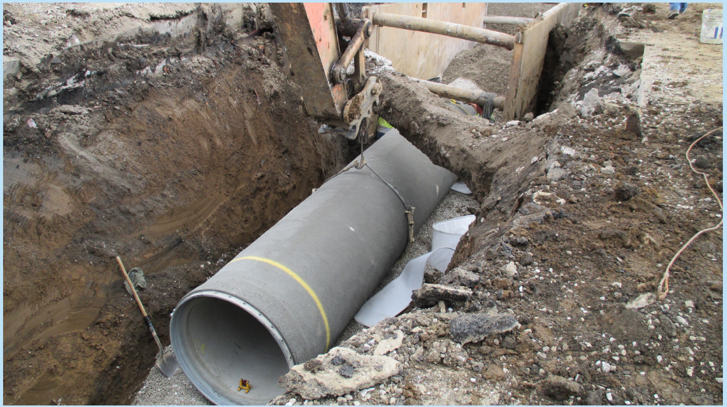
Installation of large-diameter force main with restrained joint.
