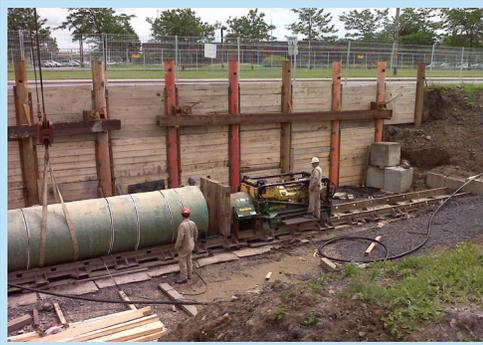
*Concrete Pressure Pipe being pushed into tunnel.*
