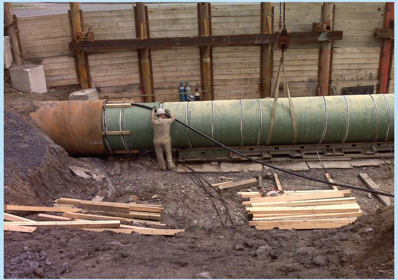
*Concrete Pressure Pipe attached to timber skids.*
