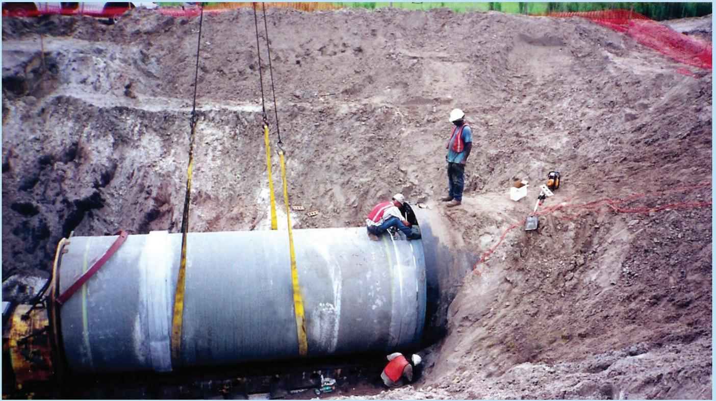
*Checking joint of Concrete Pressure Pipe before pushing pipe into tunnel.*
