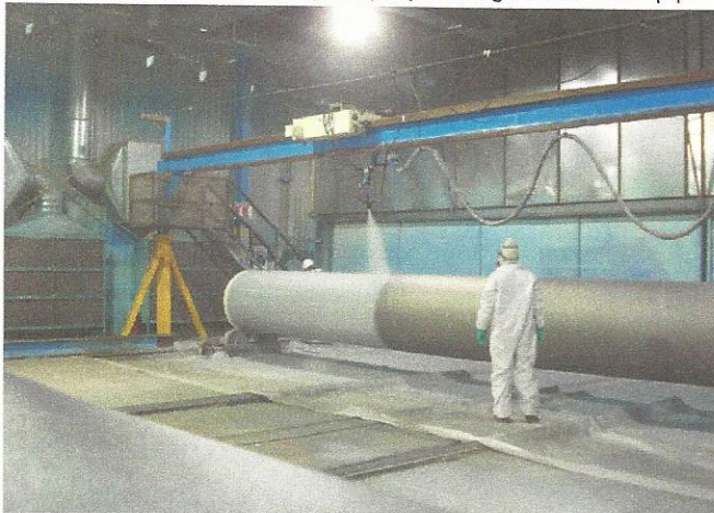
BELOW ▾ Application of liquid epoxy coating to steel water pipe.
