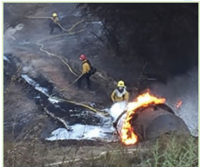
A burning HDPE culvert under Santa Barbara California Highway 101 in 2015.
