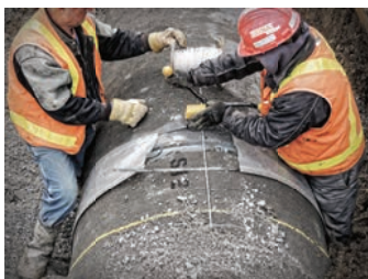
Diaper is placed around the joint and straps are tightened
