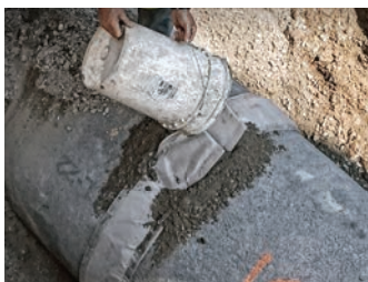
Grout is poured into the diaper into one side and then the other until the diaper is completely full
