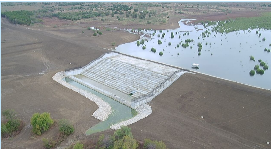
Completed NRCS dam with concrete emergency spillway built over concrete pressure pipe principal spillway installed through the dam.
