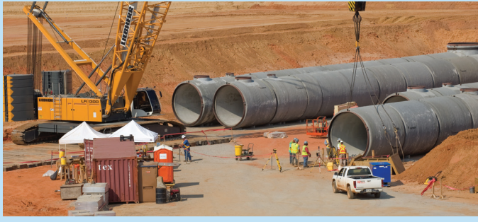
Since the early 1950s, engineers have specified Concrete Pressure Pipe and relied on its performance for cooling water pipe systems in nuclear, coal-fired and gas-fired power plants.
