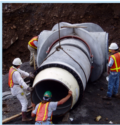
Concrete Pressure Pipe with flanged reducer is attached to cross using a joint harness assembly.
