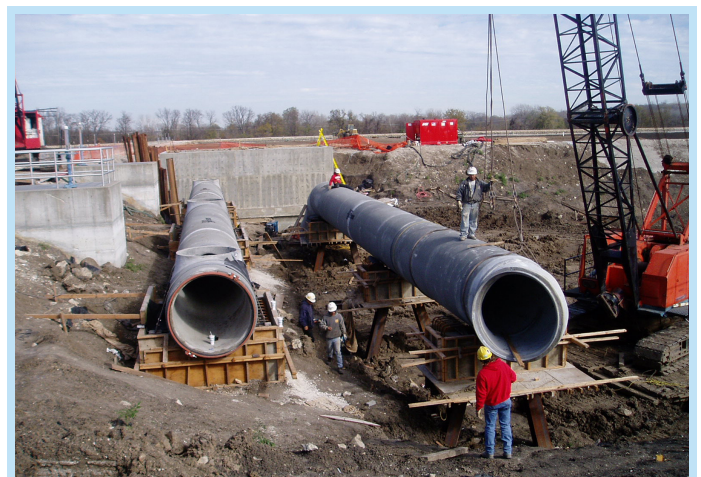
Concrete Pressure Pipe fittings provide nearly unlimited pipeline design flexibility to address treatment plant piping needs.
