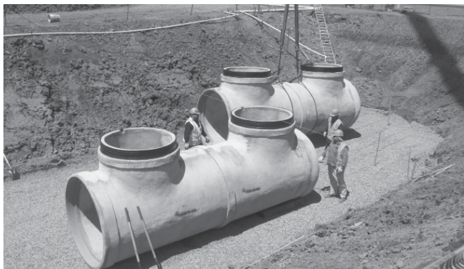
Fitting suspended vertically by sling
