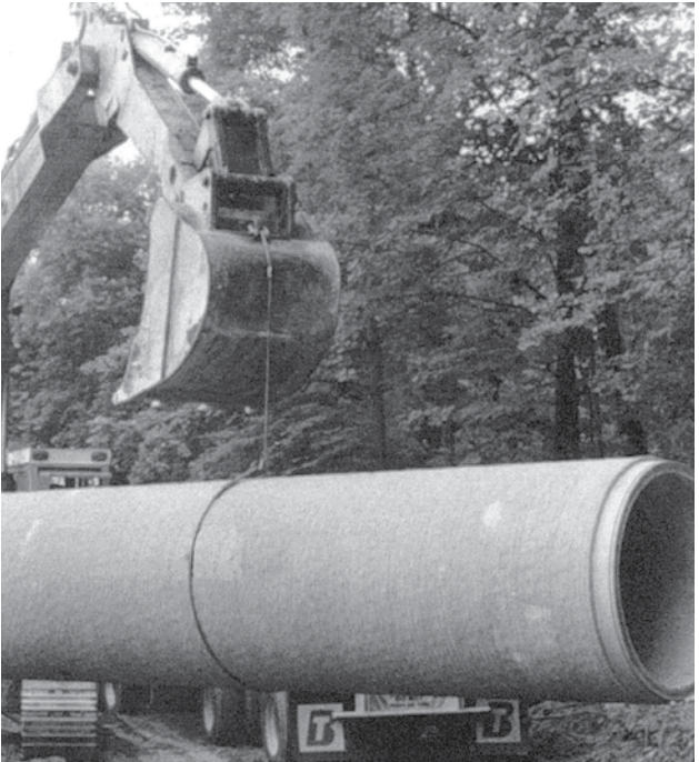
[ backhoe picking pipe up with sling ]
