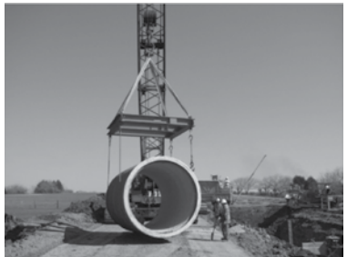
[ crane handling pipe using a lifting sling assembly ]
