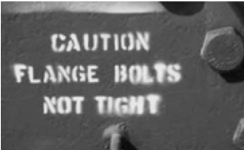
markings on a flange
