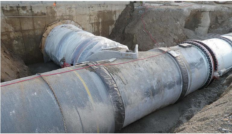
At the City of Cincinnati's Richard Miller Water Treatment Plant, more than 600 feet of 78-inch-diameter E-301 PCCP was used to reroute twin lines from the plant's GAC treatment building to a new UV facility and then to existing clear well storage.
