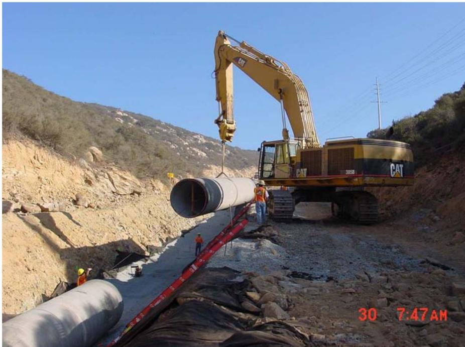
Figure 7. Installation of 66-inch diameter CCP
